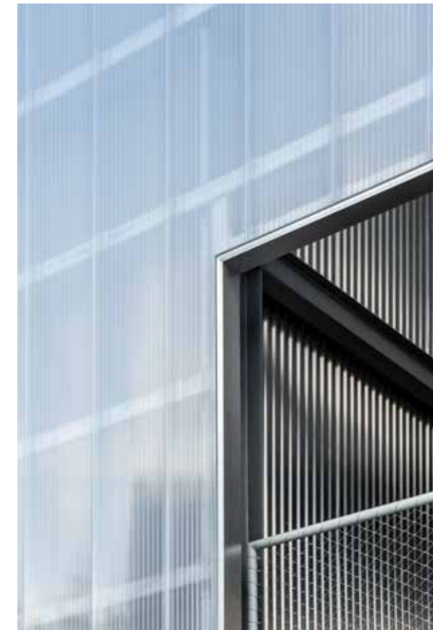
Above External material details, profiled mill finished aluminium and multi-wall polycarbonate
